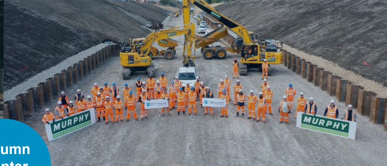
Earthworks Sectional Completions – September 2021 onwards
